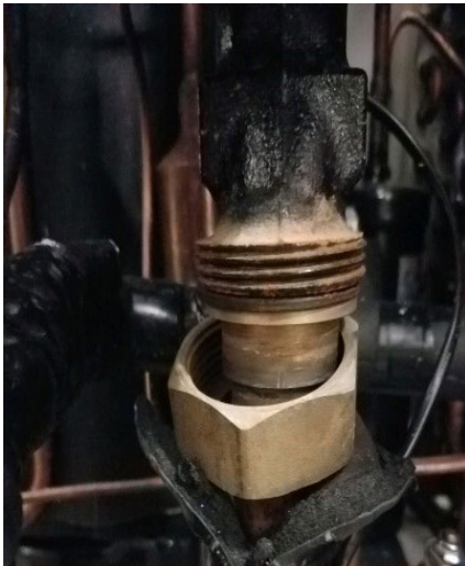
Peel back the insulation
