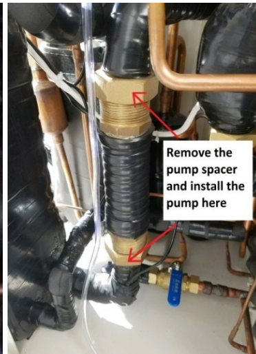
Removing the shipping spacer
