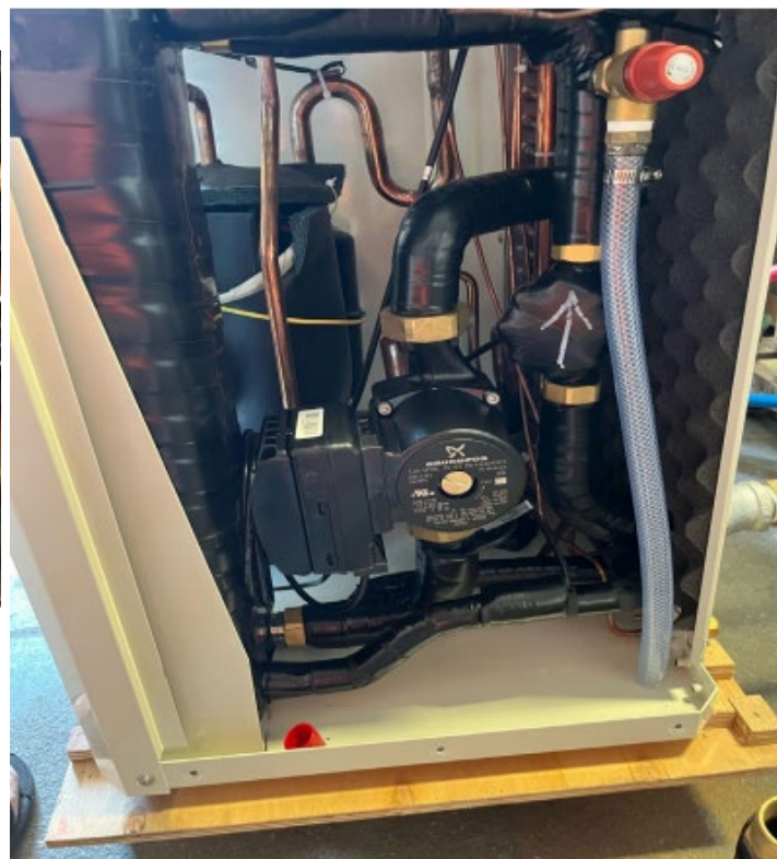
Removing the shipping spacer
