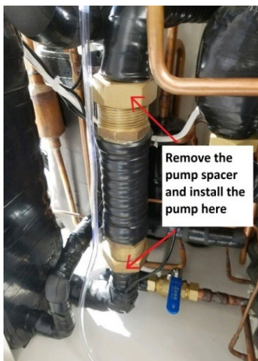
Removing the shipping spacer
