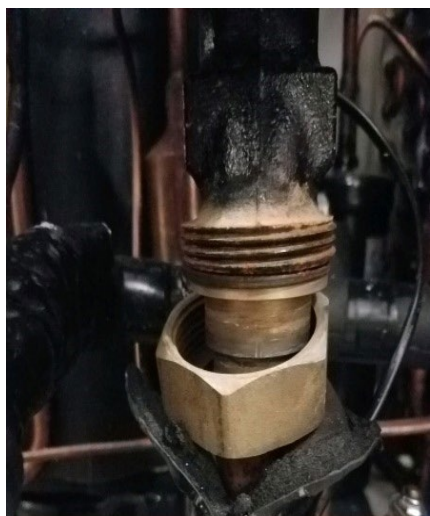
Peel back the insulation
