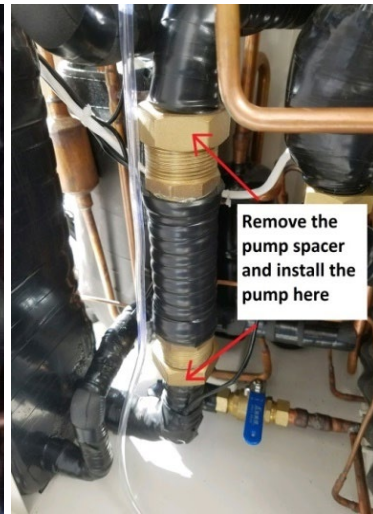
Removing the shipping spacer
