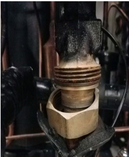
Peel back the insulation
