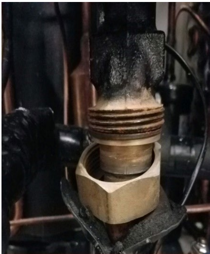
Peel back the insulation
