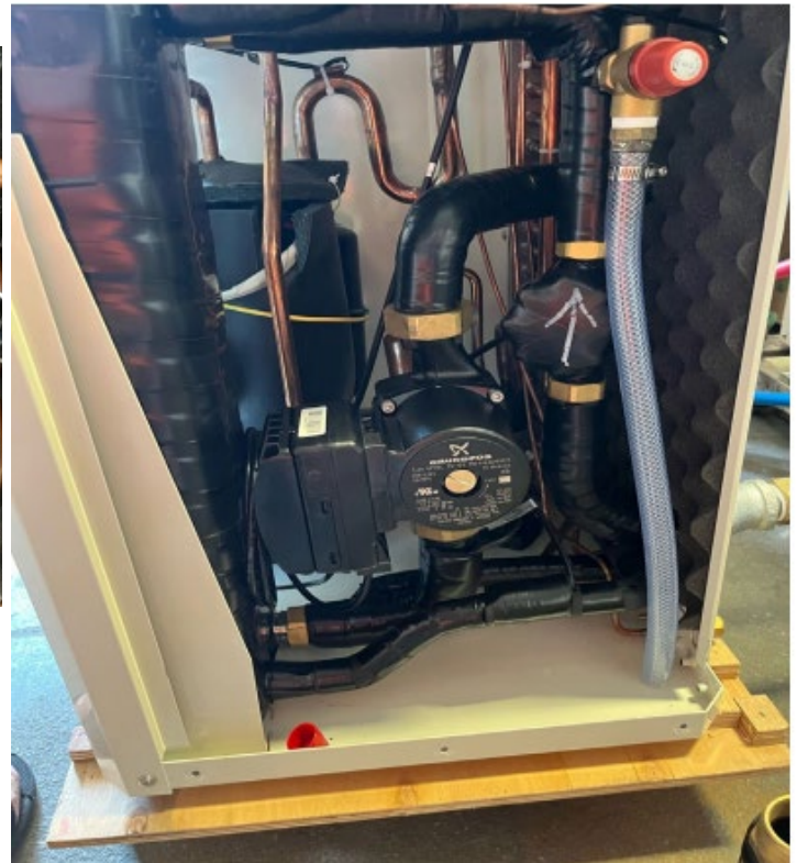
Removing the shipping spacer
