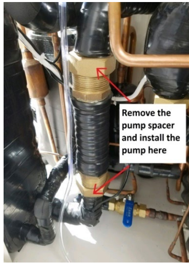
Removing the shipping spacer
