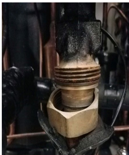
Peel back the insulation
