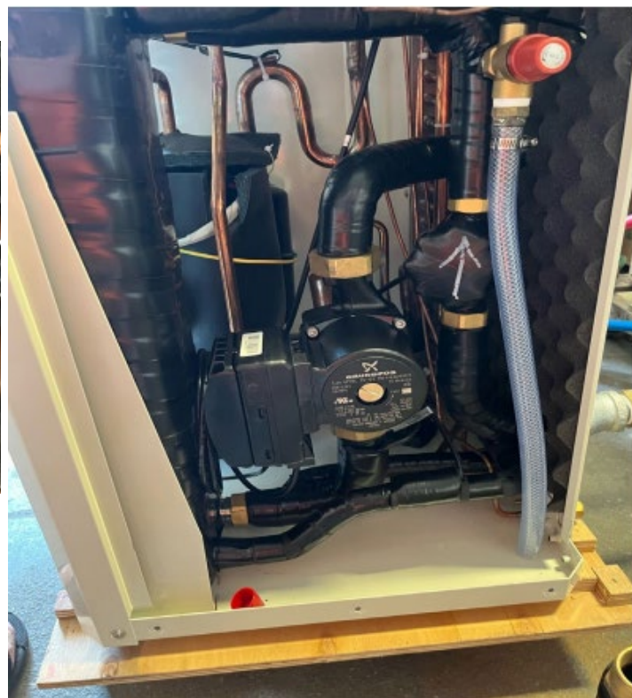
Removing the shipping spacer
