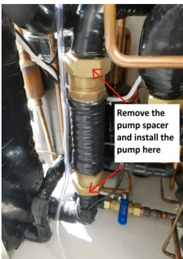
Removing the shipping spacer
