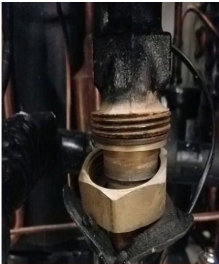
Peel back the insulation
