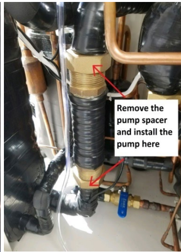
Removing the shipping spacer
