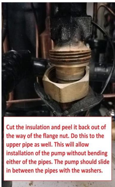
Peel back the insulation
