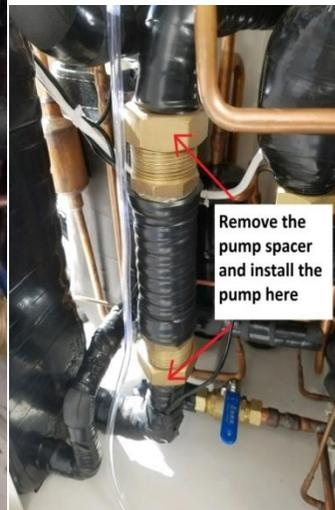
Removing the shipping spacer
