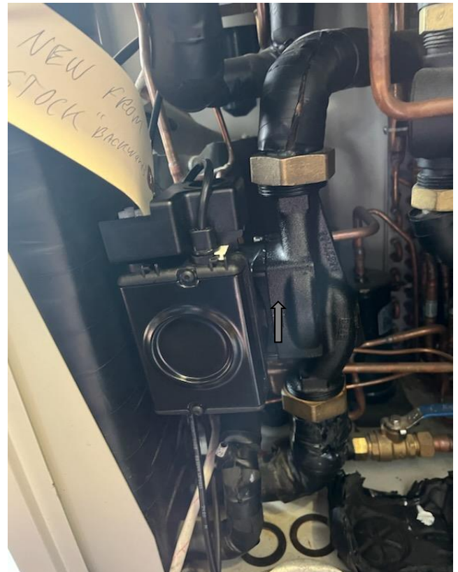
Removing the shipping spacer
