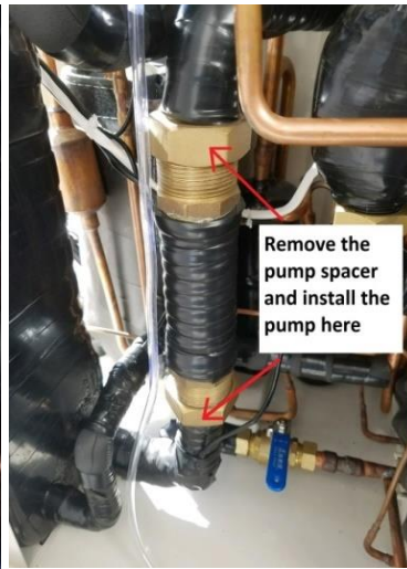
Removing the shipping spacer
