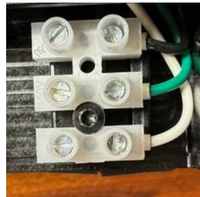
Pump Power (pump)
