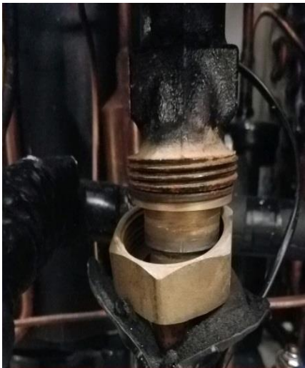
Peel back the insulation
