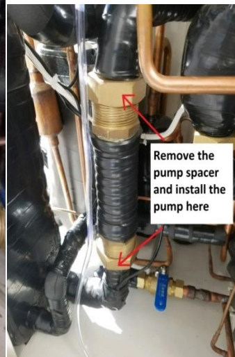
Removing the shipping spacer
