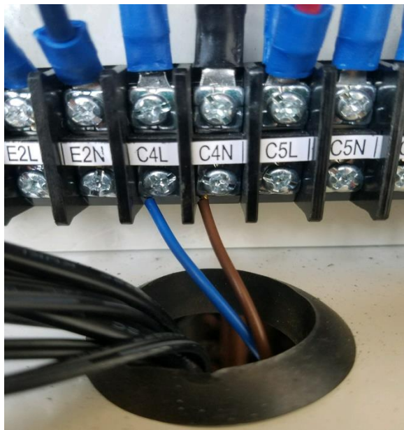
Pump power wires.
