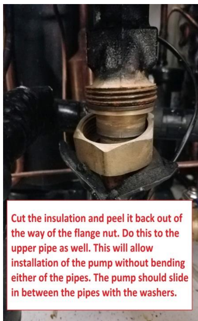
Peel back the insulation
