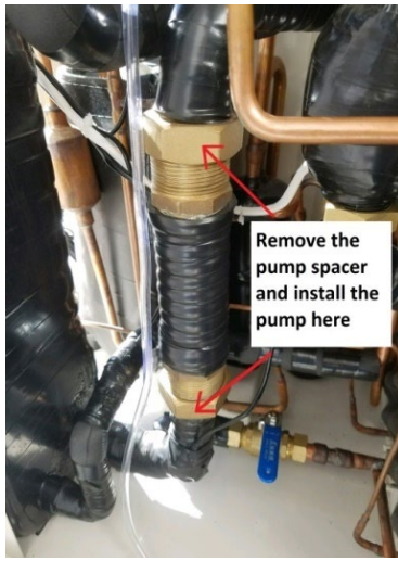
Removing the shipping spacer
