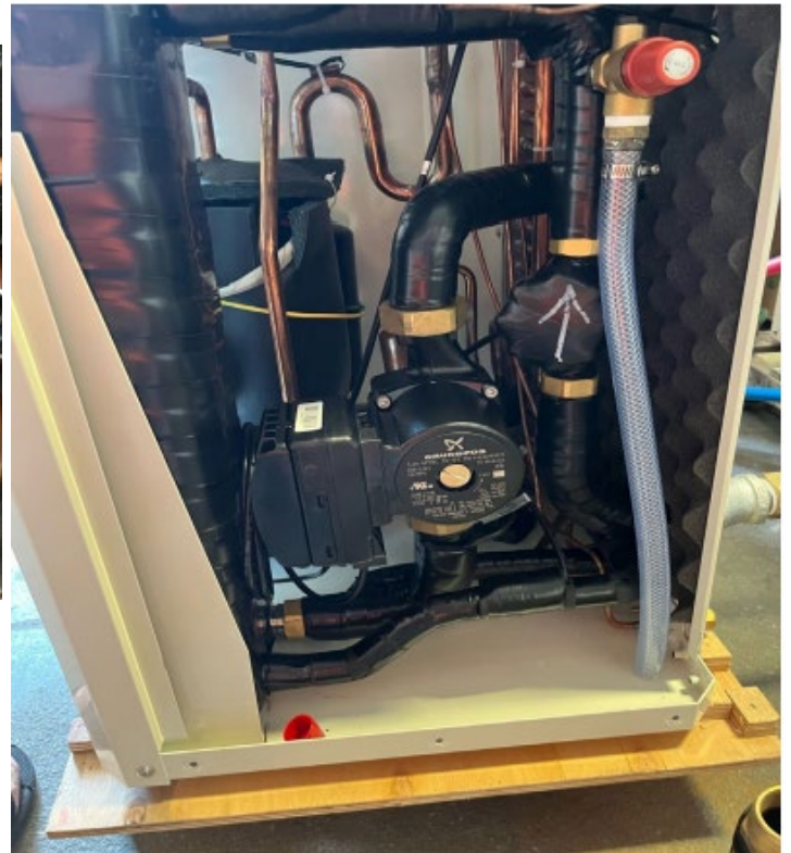
Removing the shipping spacer
