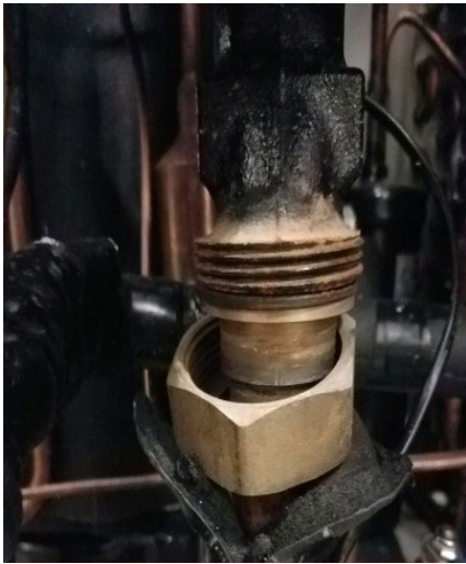
Peel back the insulation
