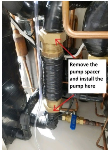
Removing the shipping spacer
